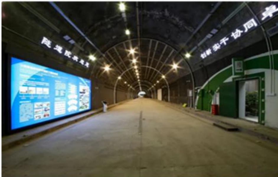
Figure 2. The final appearance of the underpass tunnel under study.
